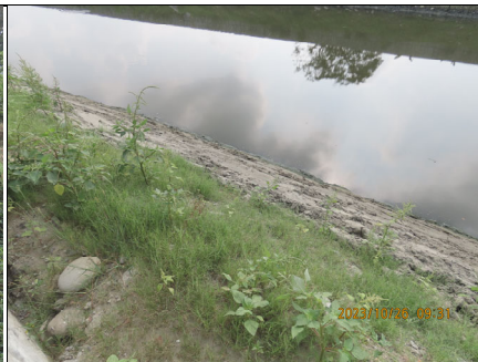
堤前土坡播撒草籽已發芽
